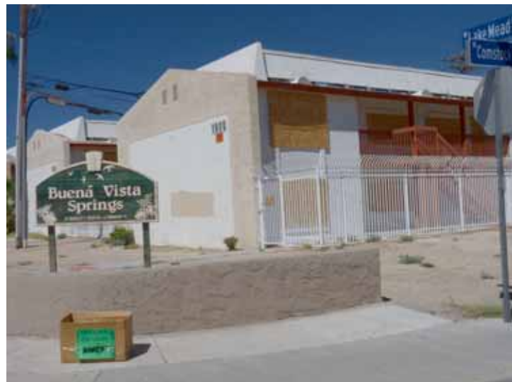
Figure 46: Boarded Up Buena Vista Springs in North Las Vegas
