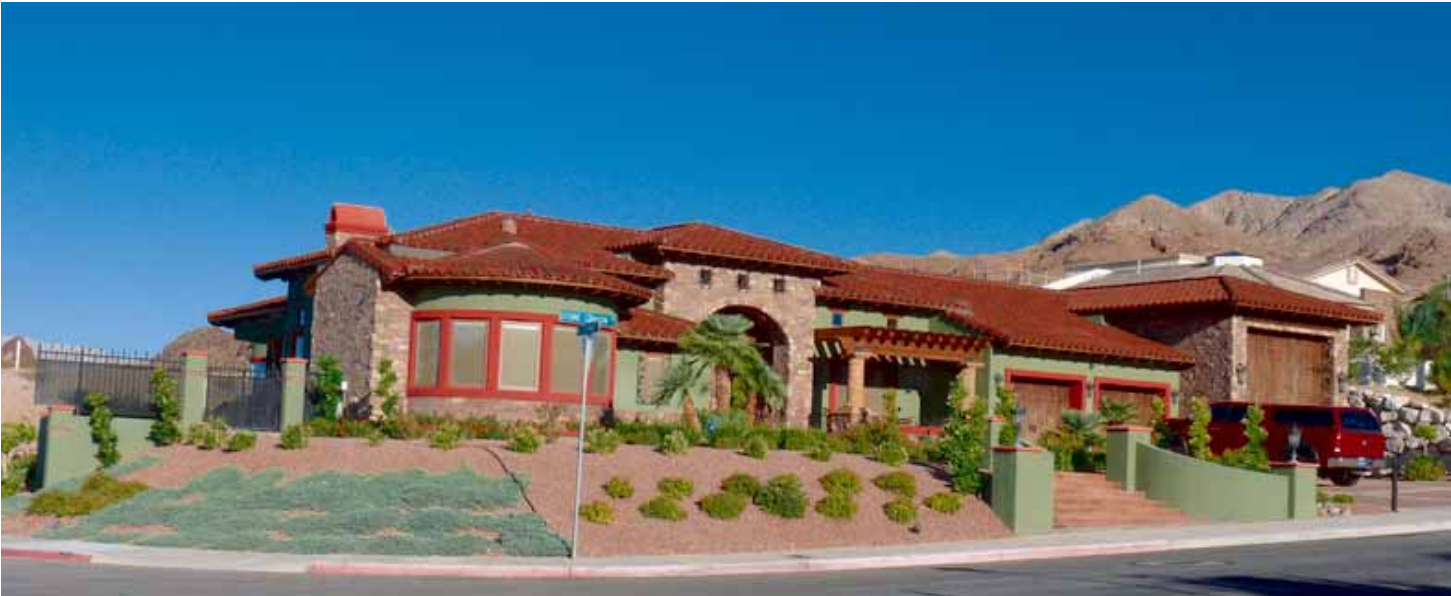
Figure 43: Higher End House in Boulder City
