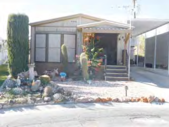
Figure 41: Mobile Home in Boulder City
