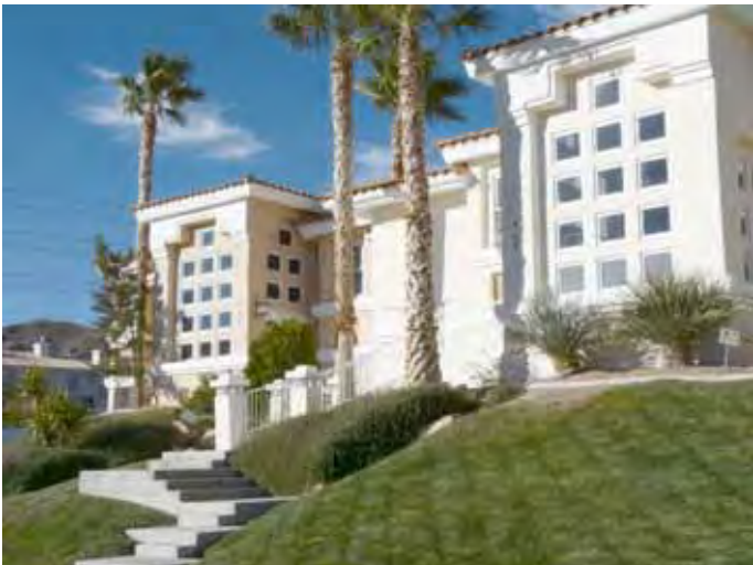
Figure 42: Condominiums in Boulder City
